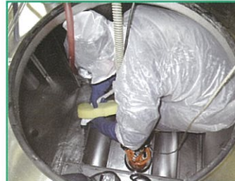
scene from cleaning the storage tank
